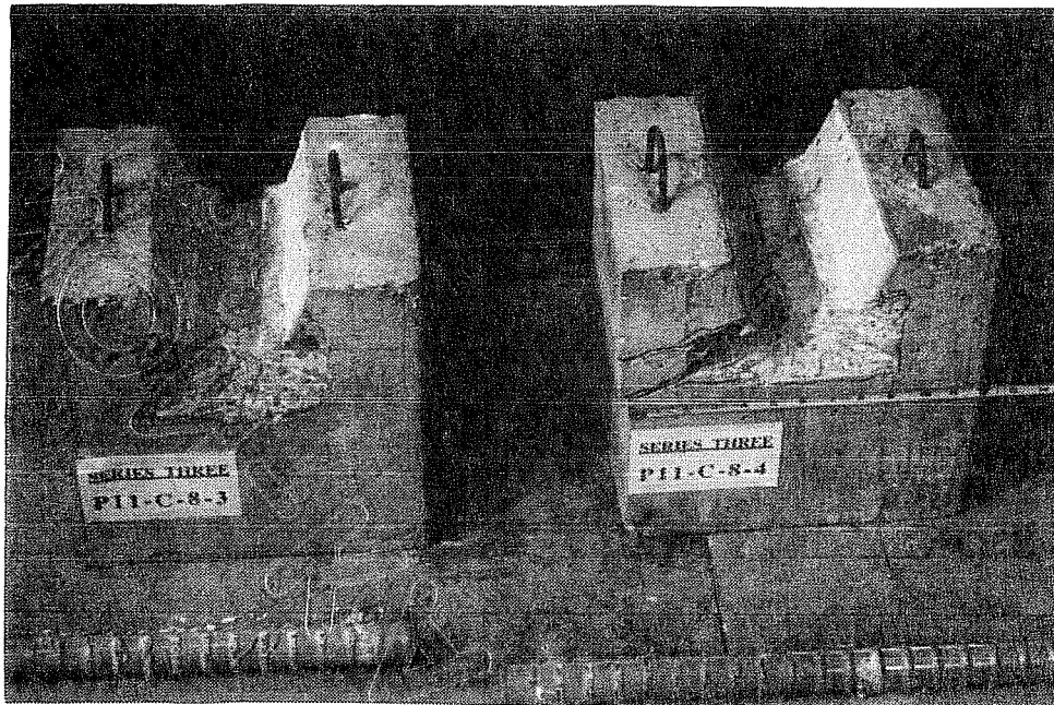
Figure 5.12 Different cracking patterns of parallel deformation pattern #11 bar Type A pullout specimens with high strength concrete.
