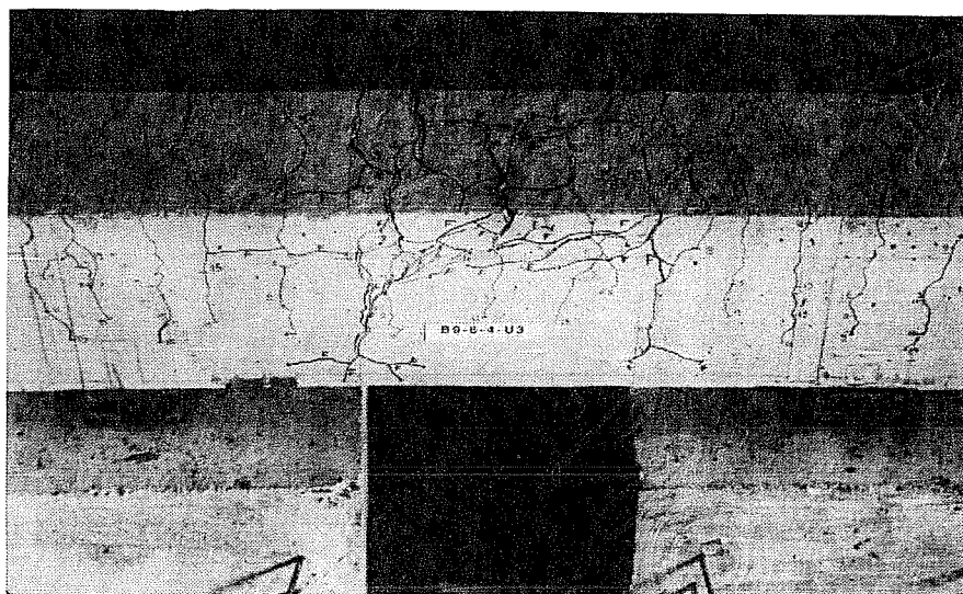
Figure 7.7 Face-and-side split failure of the uncoated bar specimen B9-6-4-U3.
